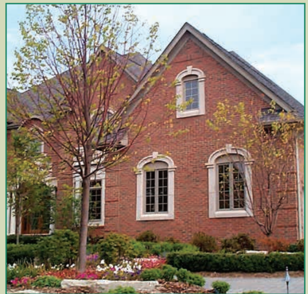
Photo above shows Spectis custom window arches with keystone.
